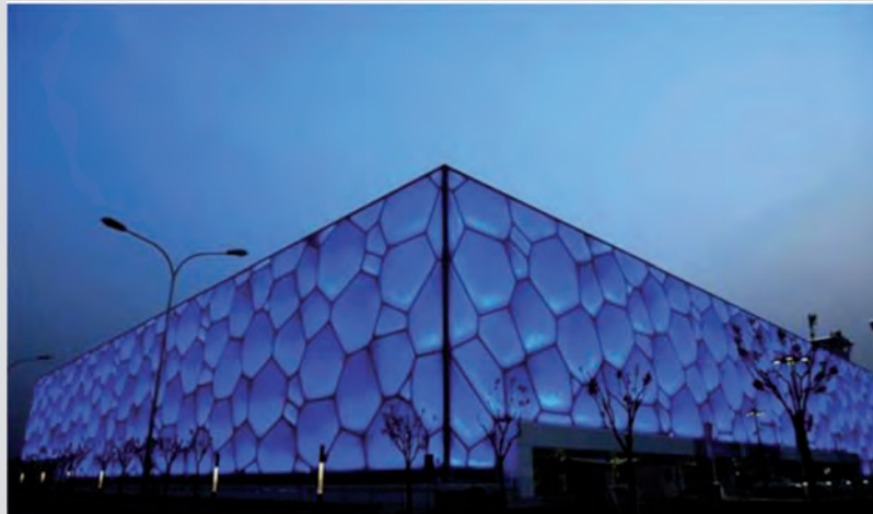
Figure 13. Innovative applications in construction: the exterior of the Beijing National Aquatics Centre, the world's largest building covered entirely by ETFE (ethylene tetrafluoroethylene)
