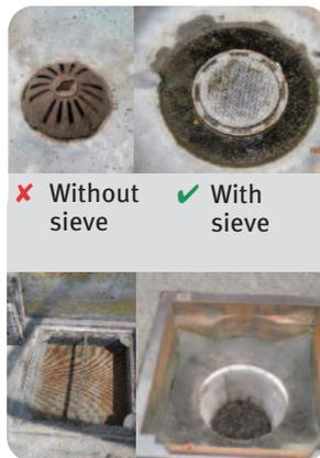
Filtration system on waste water drain:
