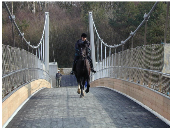
This particular bridge is designed for horses and foot traffic, but FRP full load-bearing road bridges are also being built in a similar way.
