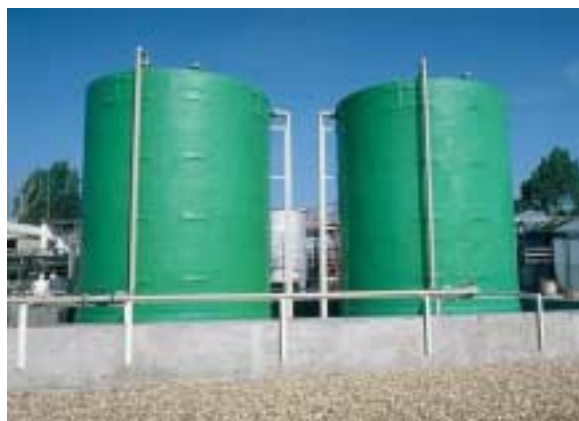
Emergency retaining pit should hold 110 % of the largest tank capacity.
