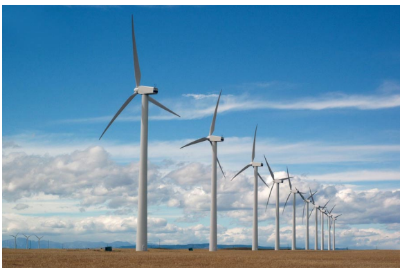
Above: Low weight and high strength makes FRP ideal for windmill blades.
