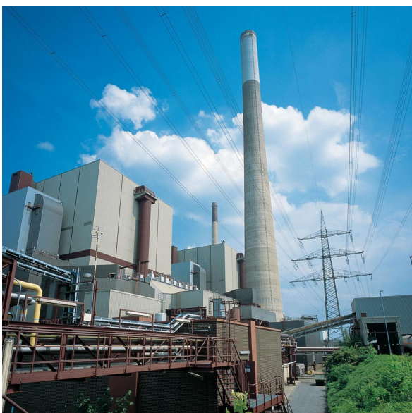
Vinyl ester based FRP was used for the inner lining of this 178m high chimney in a flu gas desulphurisation plant.
