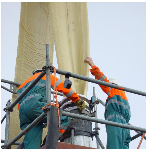
The relining process uses a composite liner that is fed into the sewer line through a convenient point such as an inspection chamber.
