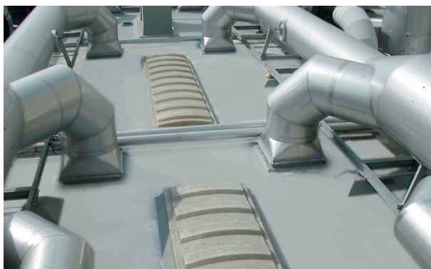
FRP composites provides a permanent waterproofing solution for flat and inclined roofs. This roof encapsulates all fitting and protrusions in a seamless waterproof membrane.
