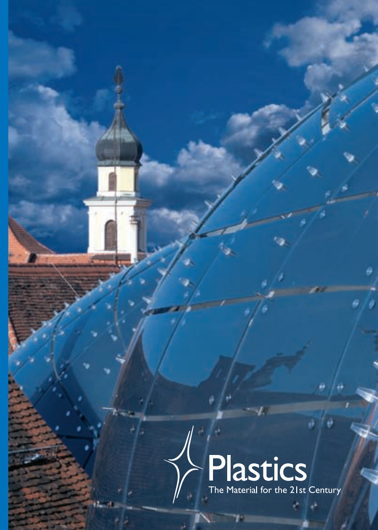
Graz, Kunsthaus. The acrylic glass facade houses a system of 930 fluorescent lamps which can be adjusted individually.
